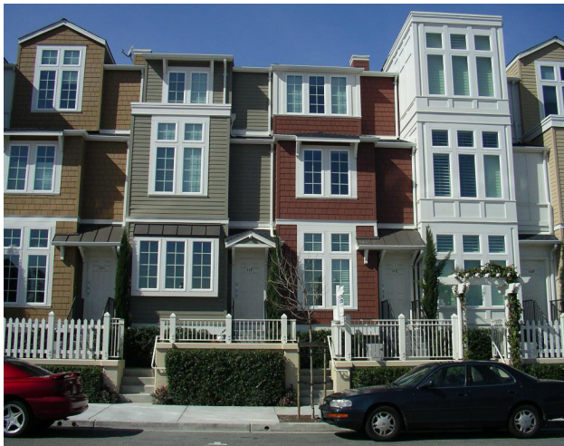
Housing types such as clustered townhomes can maintain a pedestrian scale while increasing density
