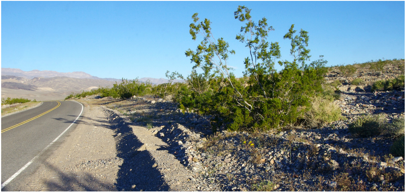
Figure 4. CA190 in Death Valley National Park looking east. Shown here are the paved road, ditch and sidecast bank with strong creosote growth. This section of road crosses an alluvial fan with many clasts and cobbles.
