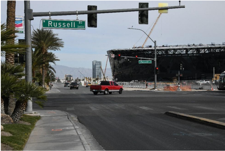
Figure 12 – Russell Road and Polaris Avenue Intersection (Looking North)
