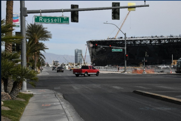
Russell Road and Polaris Avenue Intersection (Looking North)
