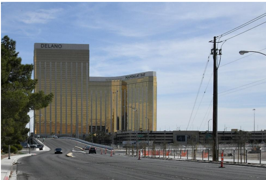
Figure 13 – Hacienda Avenue Bridge Over I-15 (Looking East)
