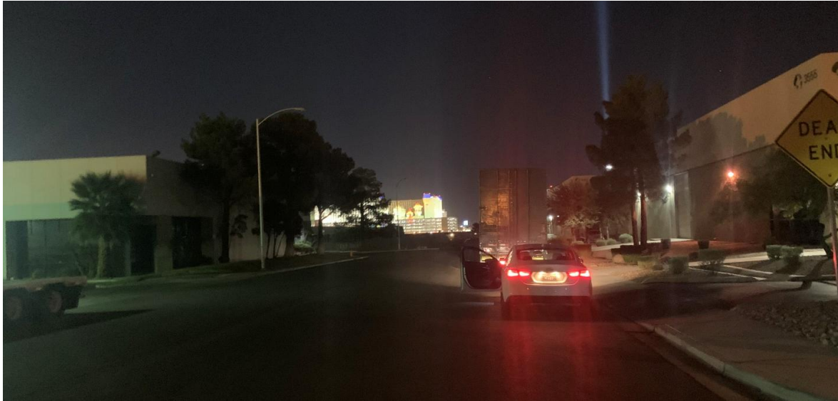
Figure 34 – Unilluminated Streetlight at Reno Avenue and Procyon Street
