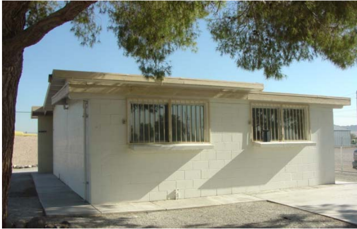
Existing restroom building.
