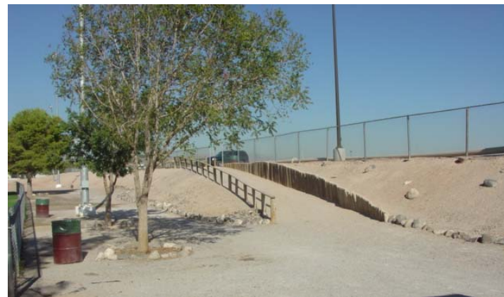
Existing ramp from Dog Fancier's Park to the north parking lot.
