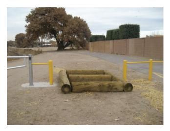
A motorized vehicle barrier that allows for equestrian passage
