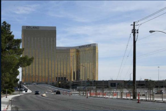
Hacienda Avenue Bridge Over I-15 (Looking East)
